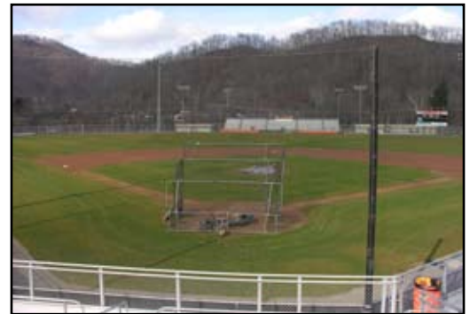
Ball field constructed by mining company for the residents of Chapmanville, W.Va.
